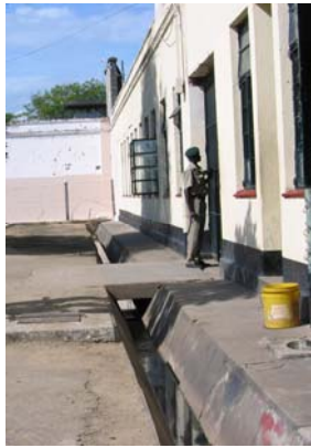
The outside room for day use The open gutters were originally designed for rain discharge (monsoon climate!) Now also "Grey water"
