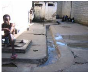
The outside room for day use The open gutters were originally designed for rain discharge (monsoon climate!) Now also "Grey water"
