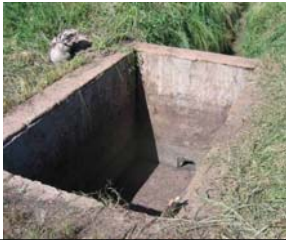
Where the sewer changes in a open discharge
