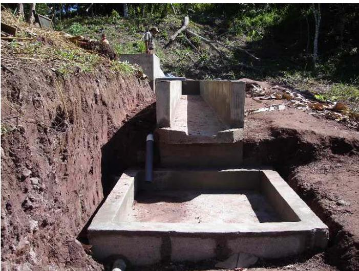
Figure 3.1: Concrete wastewater collector
