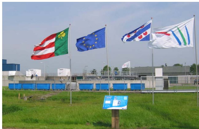
STP Grou, The Netherlands Very low loaded activated sludge (oxidation ditch)
